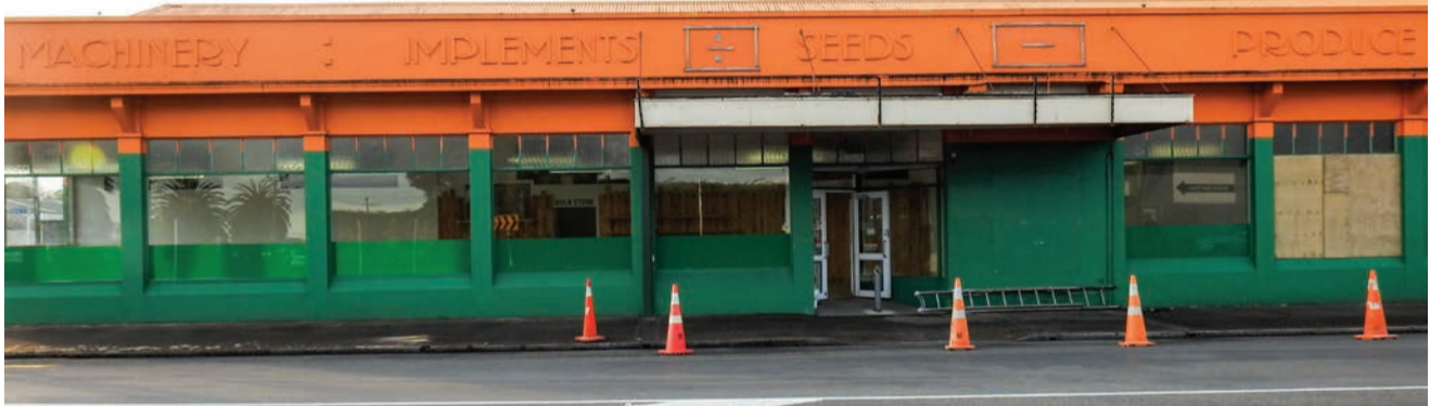
The old Farmers Co-op building which from next week will be the new home to Eltham Farm Supplies.
